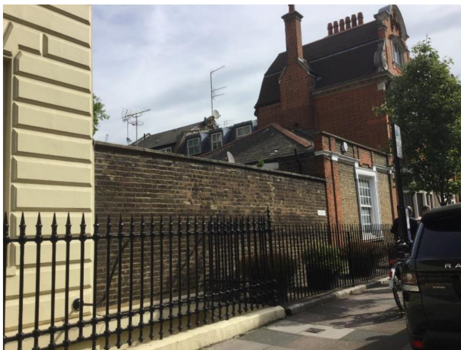
Photograph 2: Outbuilding viewed from Weymouth Street, showing elevation to be retained.
